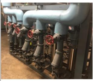
Bronze gates found in a manifold system can and should be easily exercised within a system.
